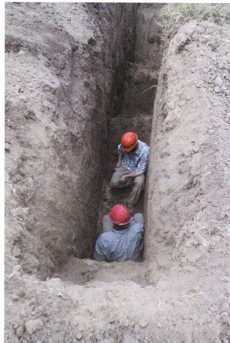
Figure 1. A backhoe dug trench exposing the stratigraphy.
