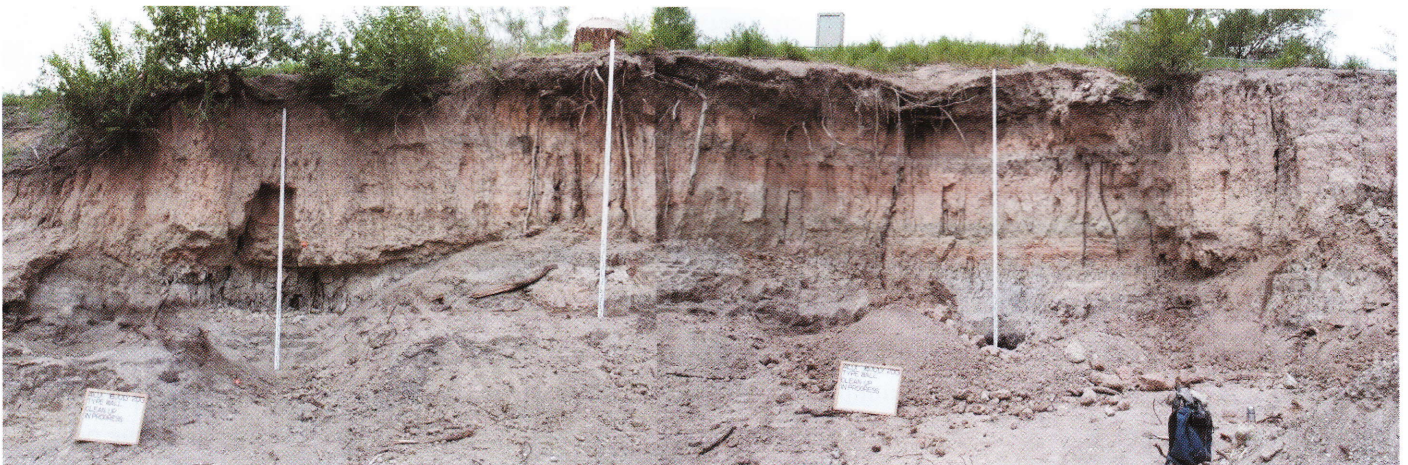
Figure 4. The type section after the bulk of the slump had been cleared away from the wall.
