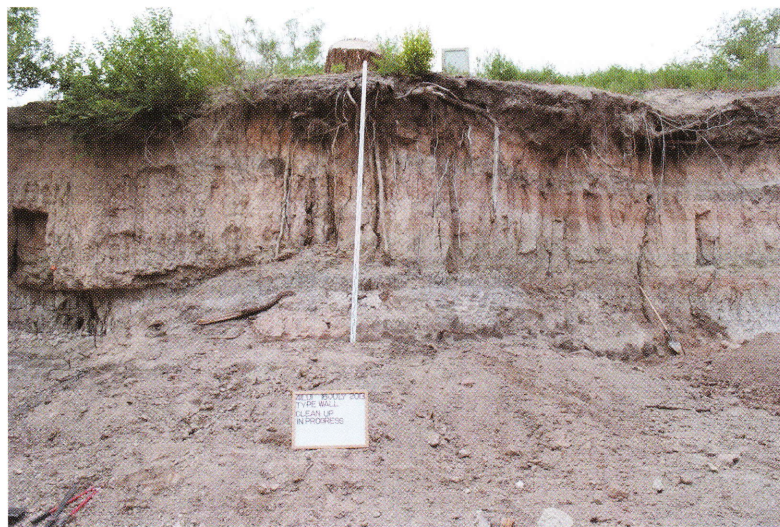
Figure 3. The stratigraphic type wall in the process of being cleared of slump.
