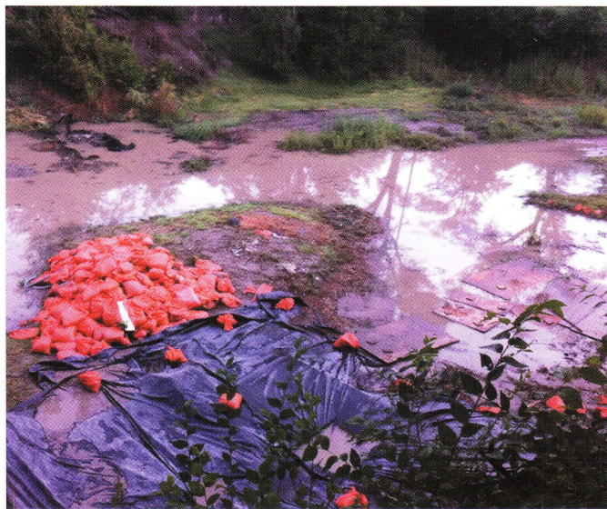
Figure 2. Flooding in Area 6, from above and toward east wall.
